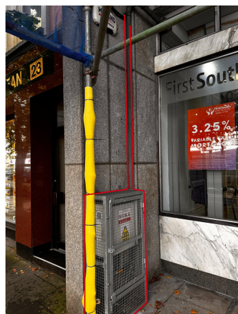
16 EXISTING GAS LINES AND PENETRATION INTO BUILDING ENVELOPE.
