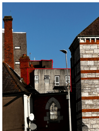
10 SOUTH FACADE OF BUILDING OBSCURED. IMAGE SHOWS REAR FIRE ESCAPE STAIRS
