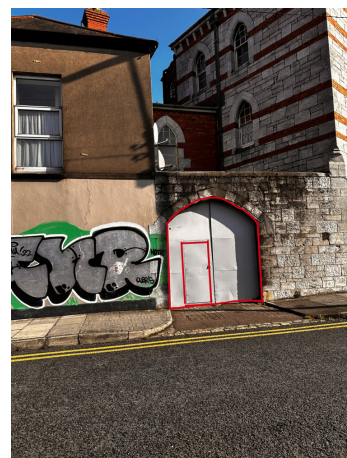
11 REAR ENTRANCE TO BE USED AS PART OF BUILDING RETROFIT. LOCATED ON FR. MATTHEW QUAY
