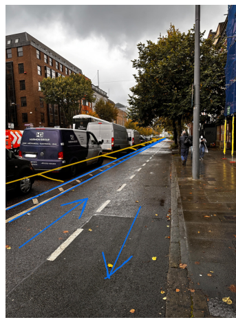
4 BICYCLE PATH SHOWN TO THE FRONT OF 24/25 S.MALL. DIRECTION OF TRAVEL INDICATED. STREET PARKING ALSO SHOWN.
